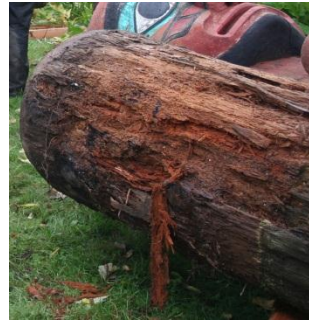
Base of column with rot damage.
